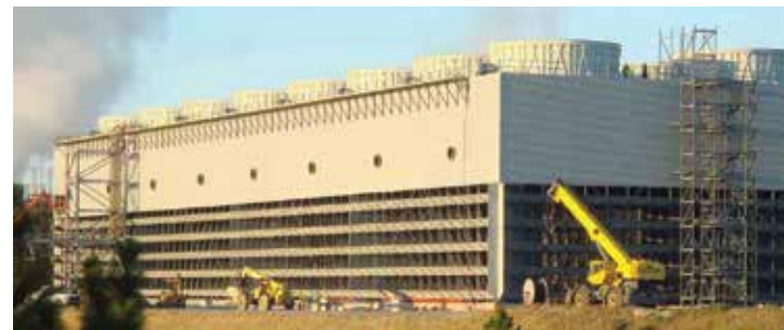
New Tower Jack Watson Power Station - Mississippi USA
