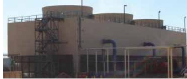
Heber South Geothermal Plant - California USA
