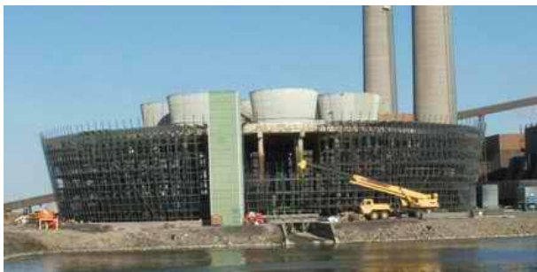
Tower Refurbishment Coal Creek Energy - North Dakota USA
