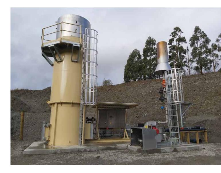
Utilising waste gas in process heating or power generation (gas engine) is a preferred method of disposal, but it is sometimes impractical due to distance from a suitable site. Gas may also need a secondary method (stand by) of disposal or the need to be load balanced with other equipment. Burning gas in a Windsor gas flare can be an excellent option in these situations.
